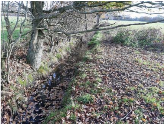
Plate 9.3: Ditch inundated with water
