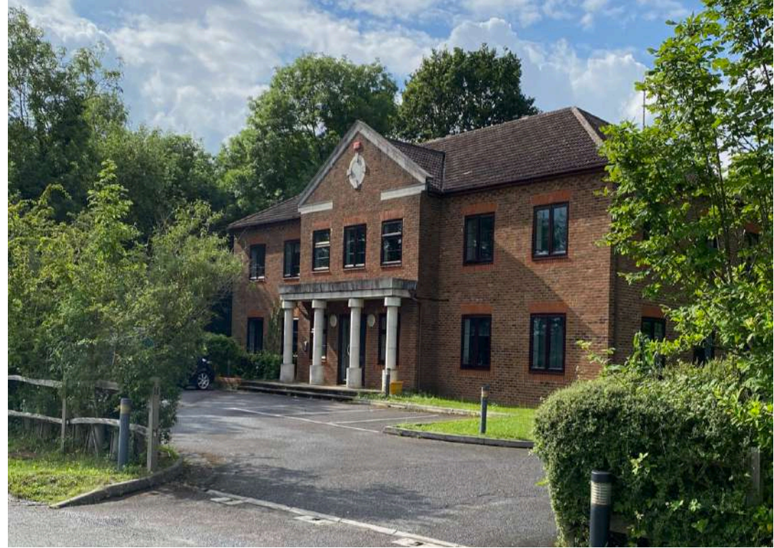
Fig 14: Fernhill House along Fernhill Road
