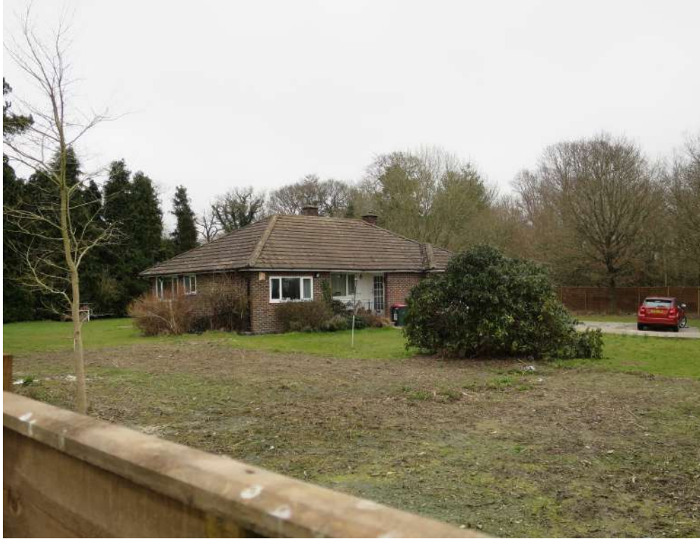
Fig 16: existing bungalow on Fernhill Road to be demolished
