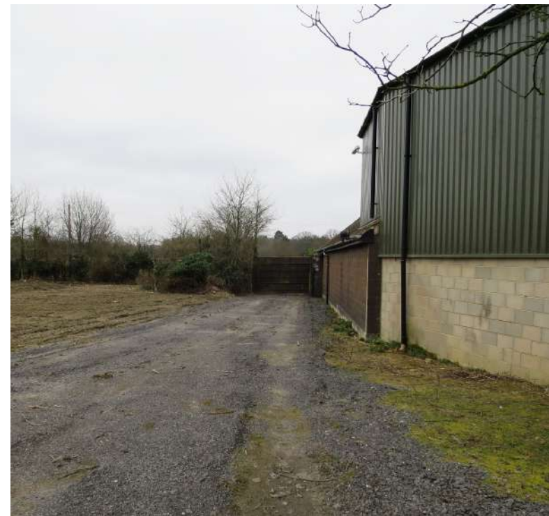
Fig 9: existing buildings on site
