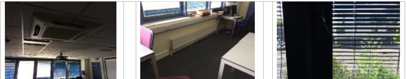
Typical classroom, with ceiling mounted split cooling unit, LTHW heating radiator. No mechanical ventilation is provided, this is achieved via openable window.
