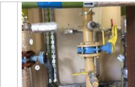
Existing VSD Htg Pumps & Gas manual shut off valve
