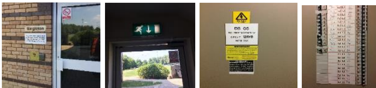
Typical security entry key pad, Fire escape sign, DB and ways
