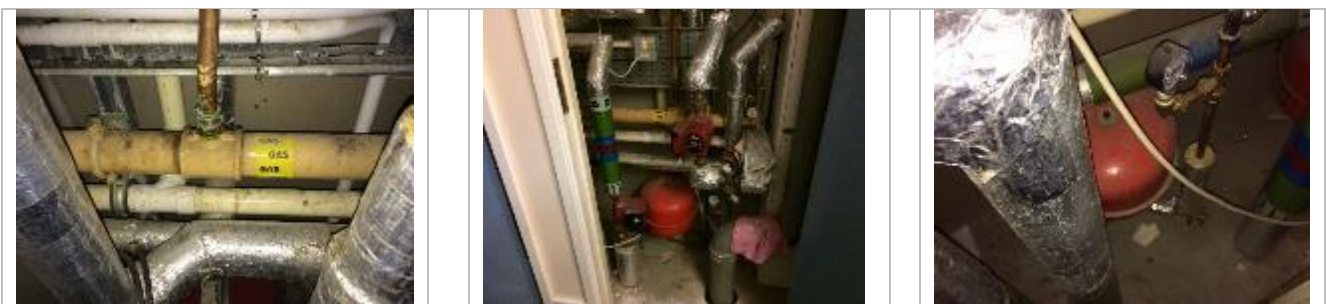
Existing gas feeding boilers, existing joint appears to be a compression fitting used, this is non-compliant under current regulations. This should be rectified as soon as possible.
