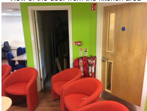
General housekeeping - Escape routes and extinguishers not kept clear, 'keep shut' cupboard left open.
