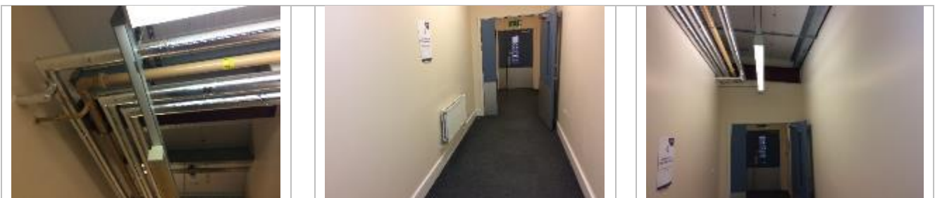
Existing gas feeding boilers, existing joint appears to be a compression fitting used, this is non-compliant under current regulations. This should be rectified as soon as possible.
