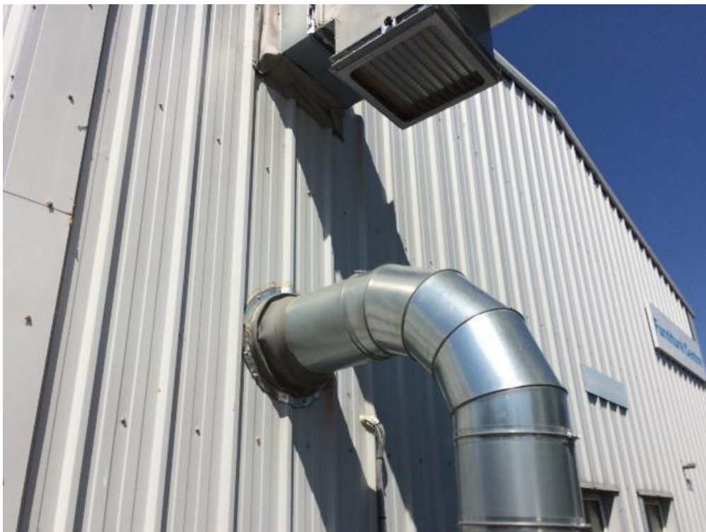
Cleaned air and additional Fresh air is the re-supplied to the workshop.
