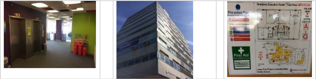
Lift lobby and external areas.
