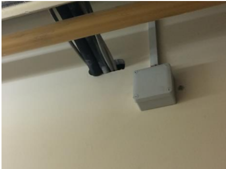
Compartmentation breaches
