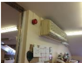
Comfort cooling wall hung split unit
