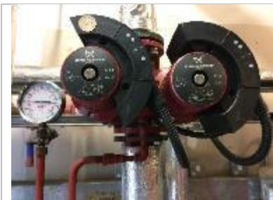
Existing VSD Htg Pumps & Gas manual shut off valve
