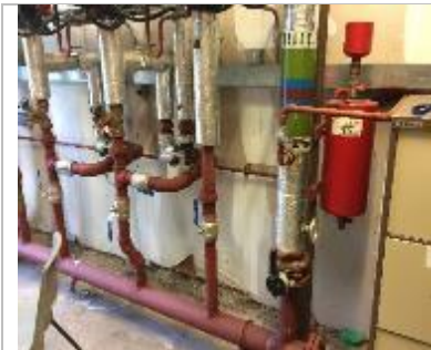
Existing LTHW header & 3 port valve
