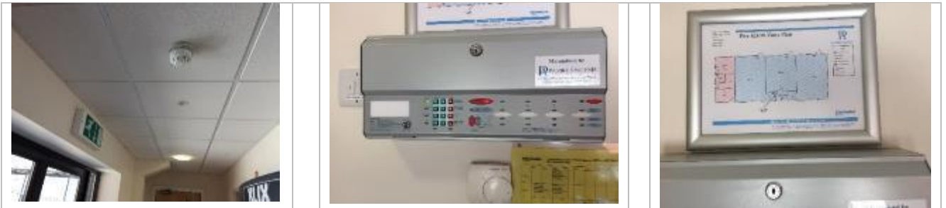
Typical PIR and FA detector, FA panel and zone plan
