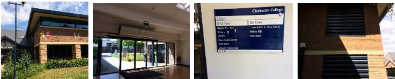
E Block main entrance and Chiller plant louvres
