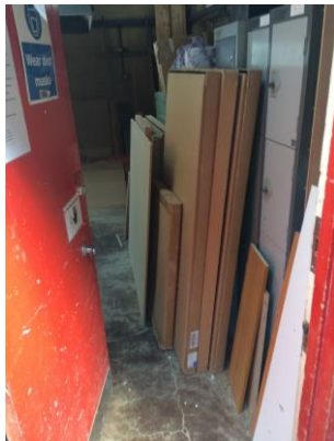
Obstructed escape routes leading to partially blocked final exit doors
