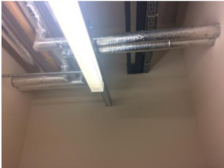
Compartmentation breaches
