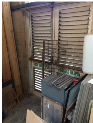
Obstructed escape routes leading to partially blocked final exit doors
