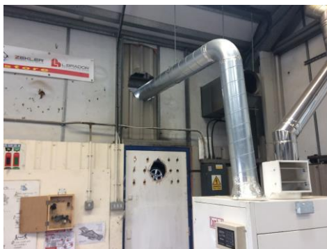
No compartmentation between workshops
