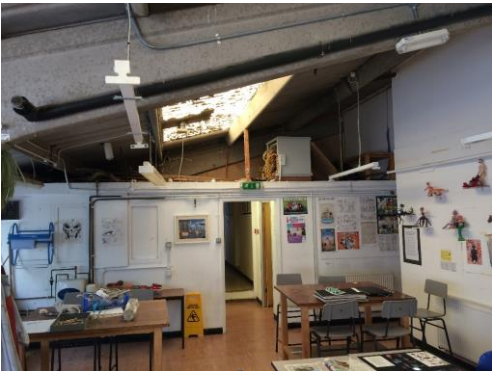
Example of first floor general condition
