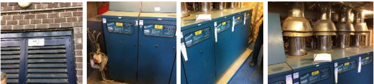
Existing Gas fired boilers & Flues
