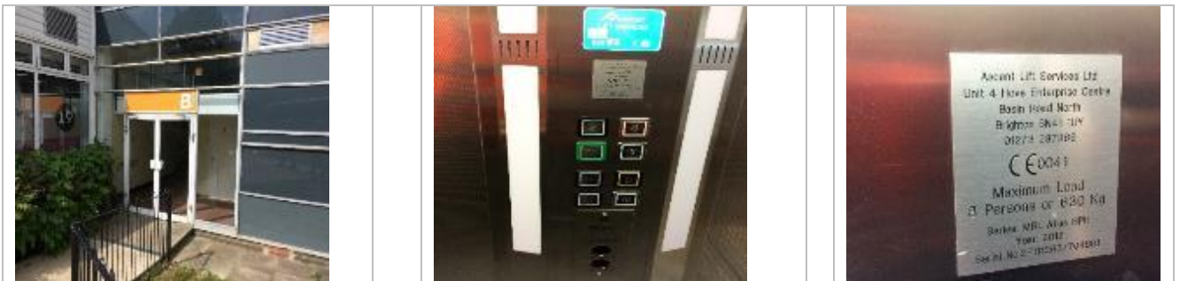
Block B, Lift.
