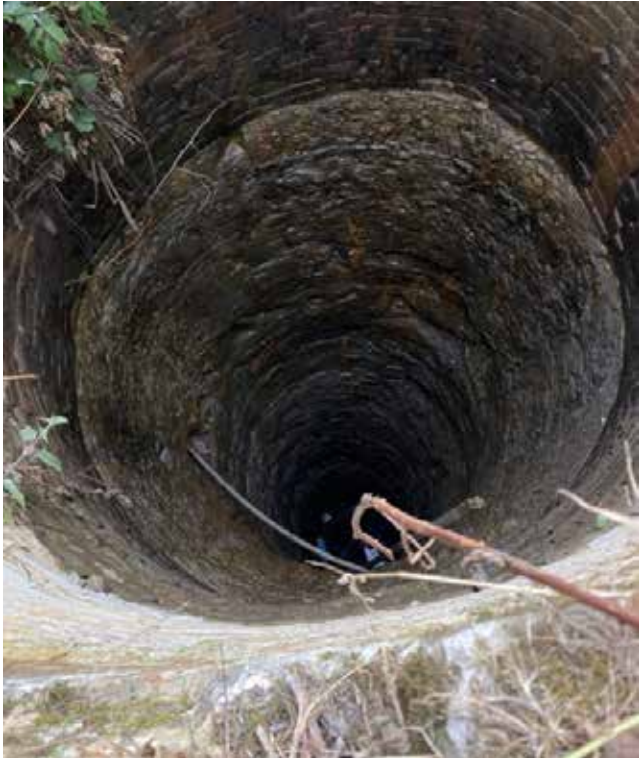
Fig 35: existing well on site
