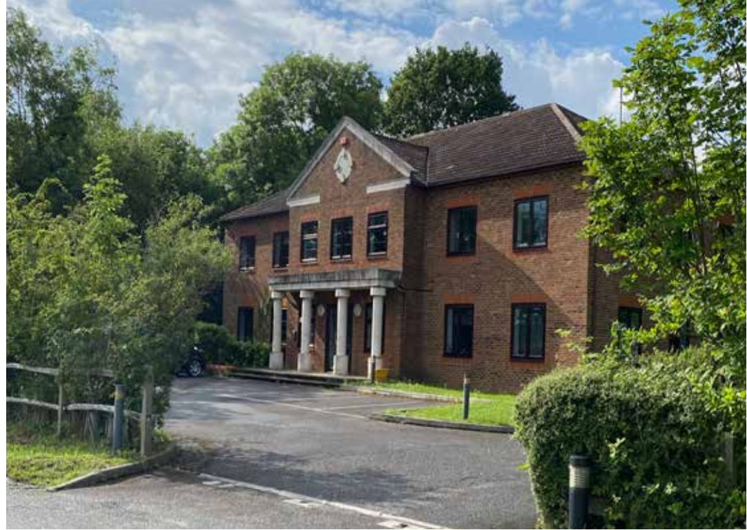
Fig 14: Fernhill House along Fernhill Road
