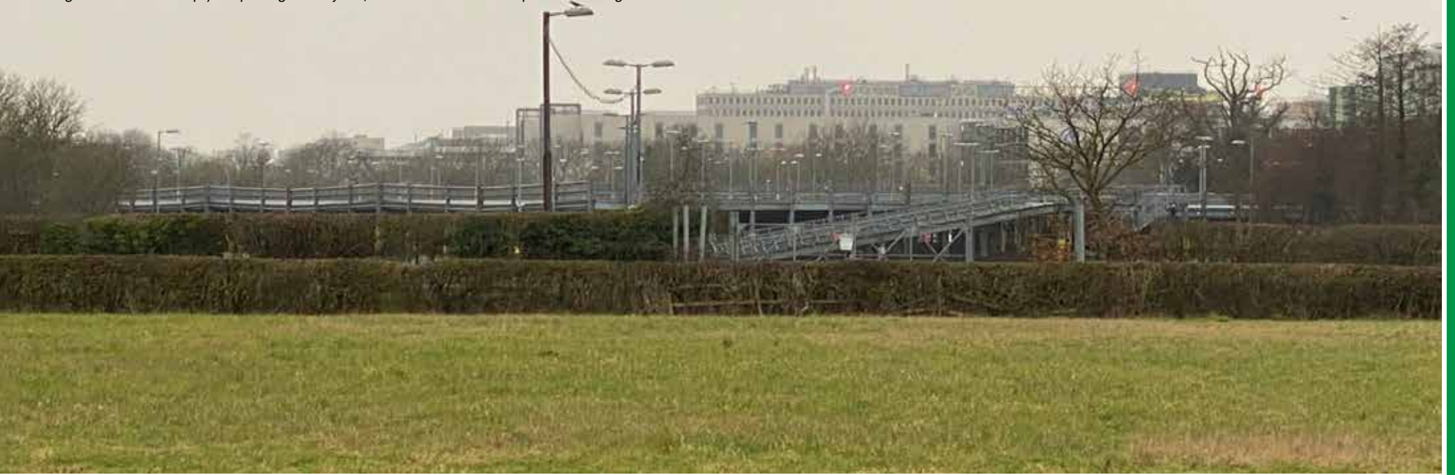
Fig 20: the site with empty Car parking and major infrastructure at Gatwick airport in the background
