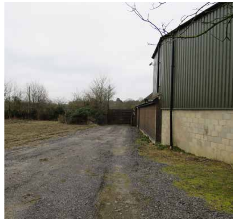
Fig 9: existing buildings on site
